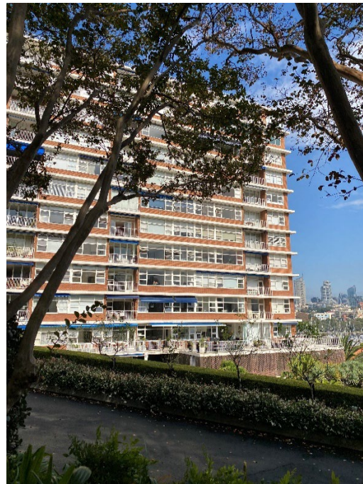
Figure 2 Glenhurst Gardens, Darling Point, completed just one year after The Gateway, was also a notable early project that utilised the lift-slab construction methodology. (Source: GML 2024)
